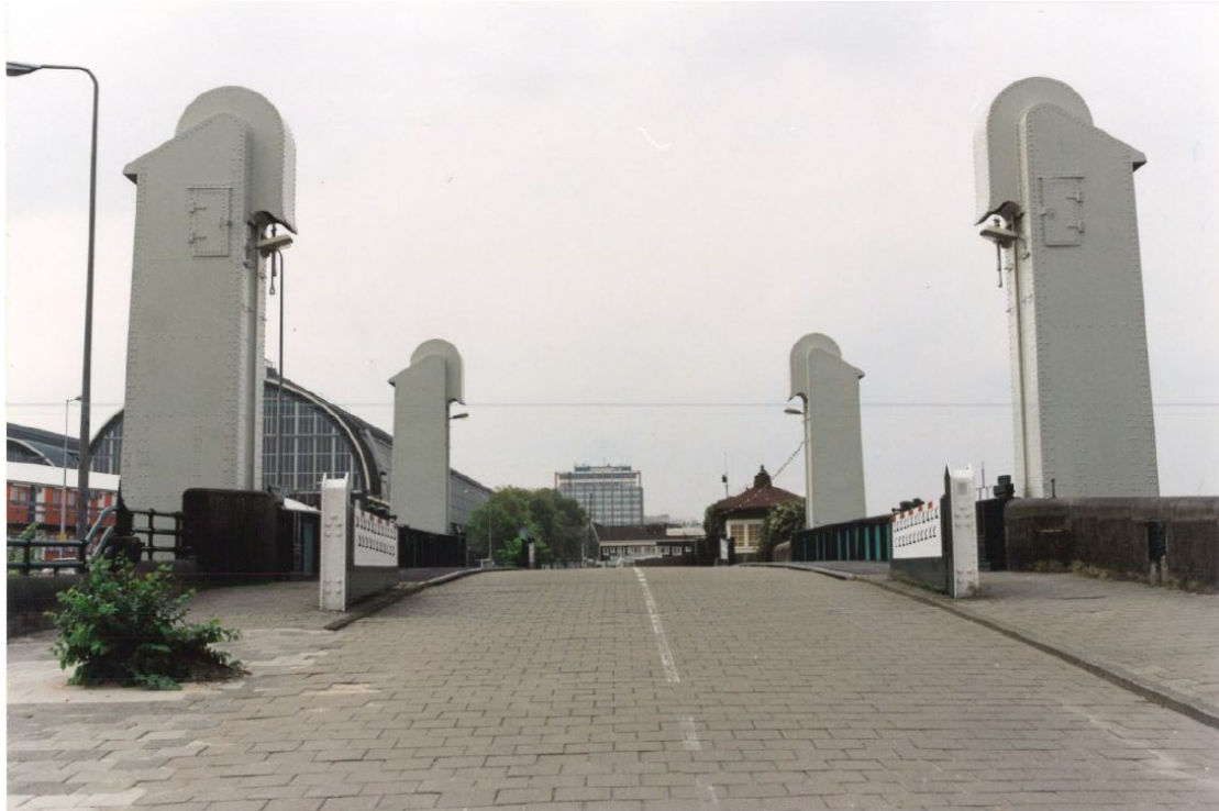
Fig. 2. Bridge as pedestrian and bicycle bridge in 2000.
