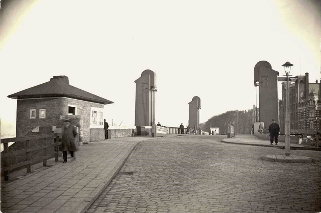
Fig. 1. Bridge at its original location
